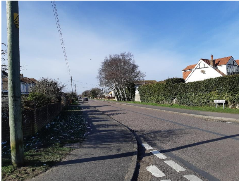
Figure 3. View of the site facing west along Queens Road
